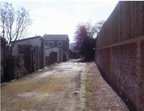
3 Side view of the wall and fences adjacent to complainants' properties
